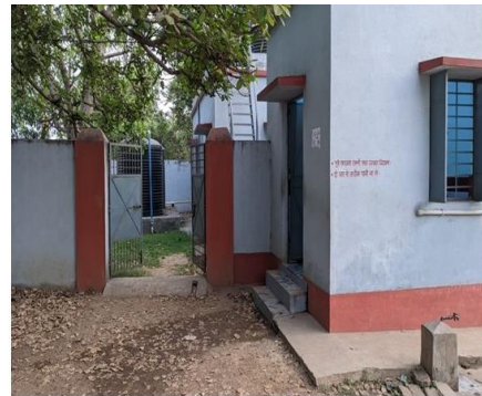
R.O Plant at Regional Hospital Chora
